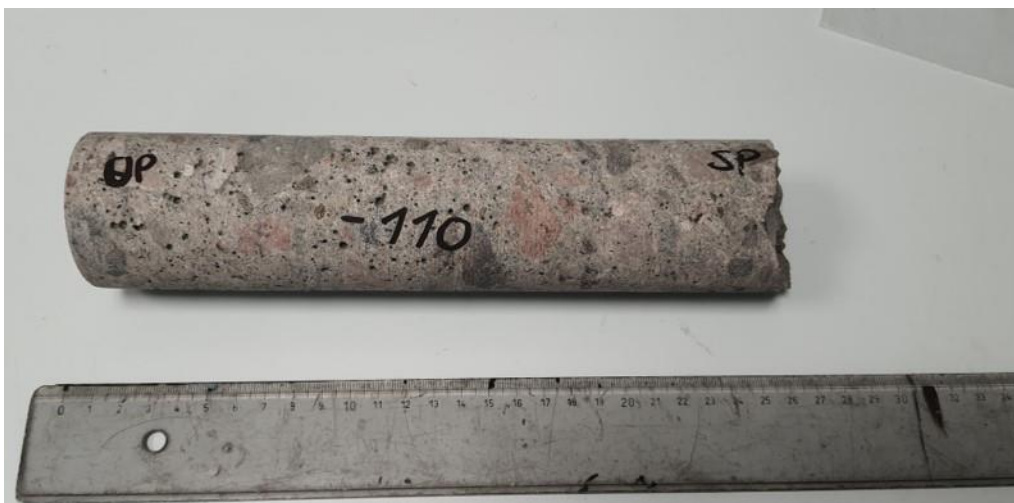
Figure 1 Photo of the LILW repository basin concrete sample core LO110.
