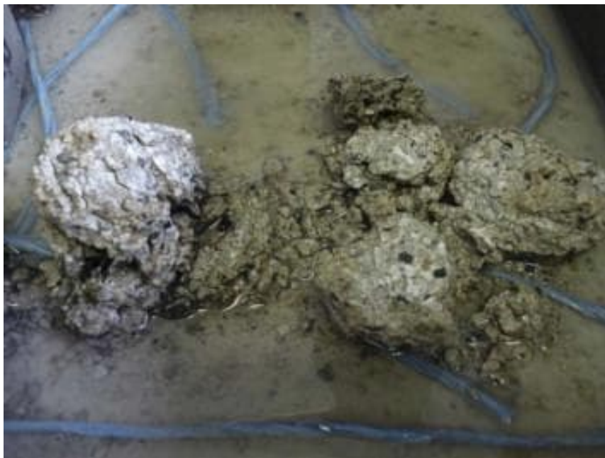
Figure 24: Concrete samples showing thaumasite formation [50].
